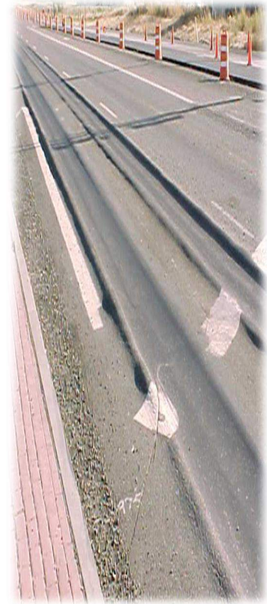
Modified asphalt mixture with crumb rubber and 50% RAP
